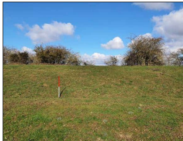
Plate 16: Sea Bank at Kirton Drain
